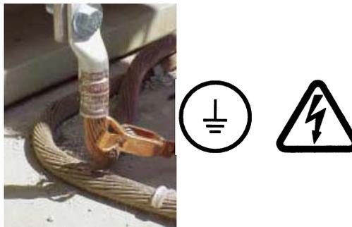
*Figure 2.1 Connecting Safety Ground to Transformer*
