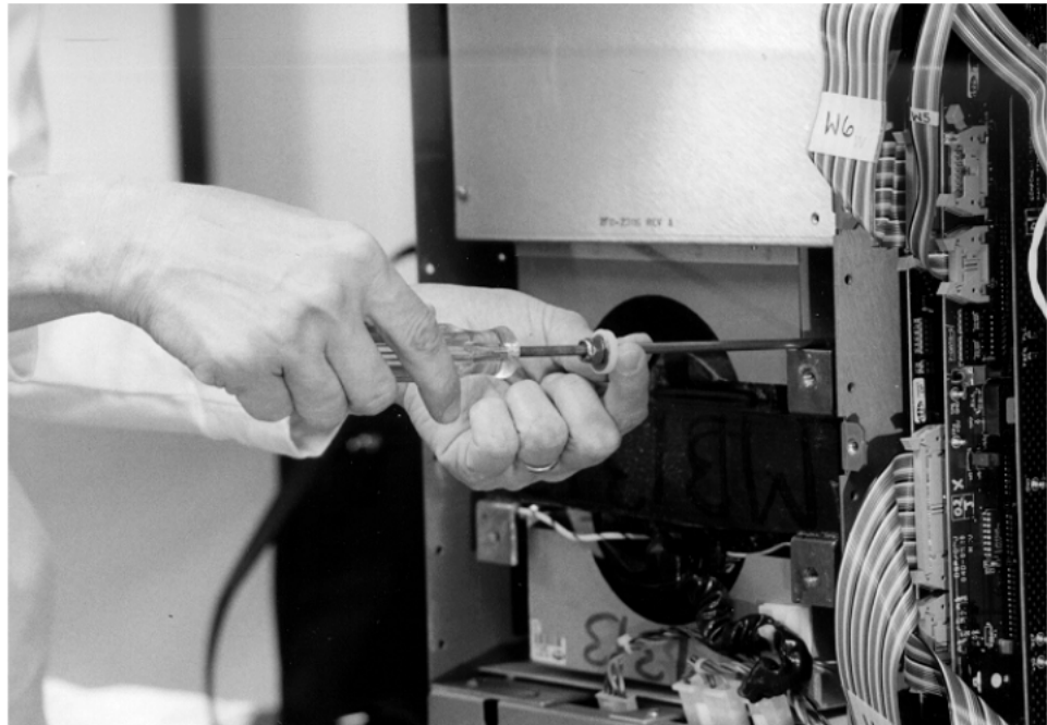
Figure 4.49 Guiding the Transformer Mounting Nuts into Position
