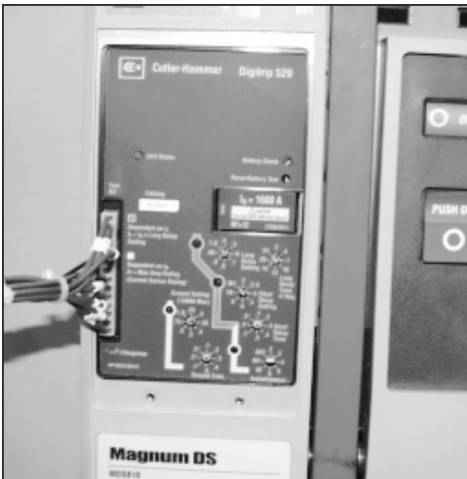
Figure 4. Trip Unit Face Plate Showing Test Port Connection
