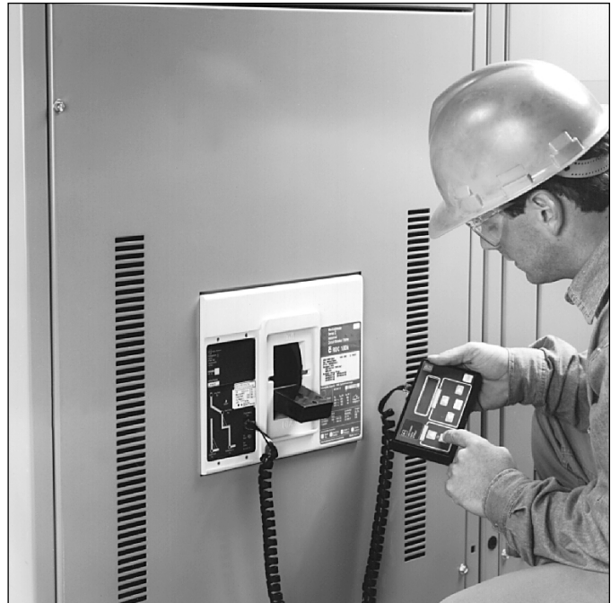
Figure 1-1 Hand Held Programmer in Use with Series C R-Frame Circuit Breaker
