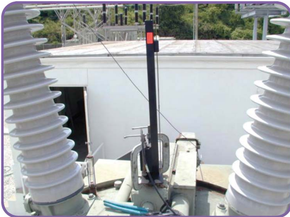
Figure 26. Linear Transducer on an OCB
