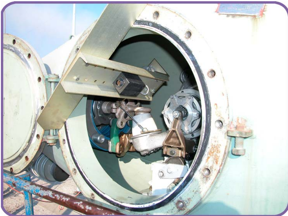
Figure 29. Westinghouse SFA Transducer Installation
