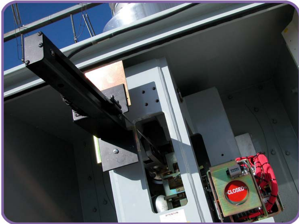
Figure 33. Linear Transducer on Mitsubishi 500-SFMT
