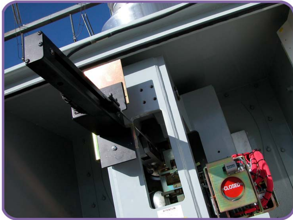
Figure 29. Linear Transducer on Mitsubishi 500-SFMT
