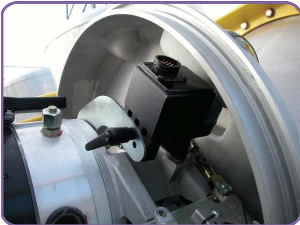
Figure 24. Rotary Transducer on ABB HMB Mech
