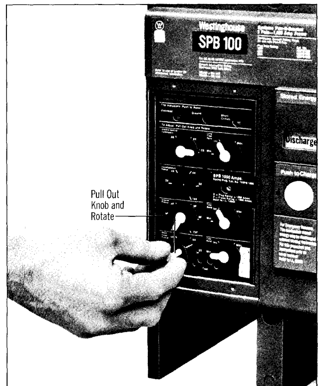
Fig. 5 Changing Trip Position Setting on Pow-R Trip 7 Trip Device
